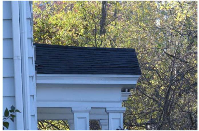
(left) Look closely at the roof structure. By not tying this porch roof together across the front, the resulting effects have pushed the supports outward.
