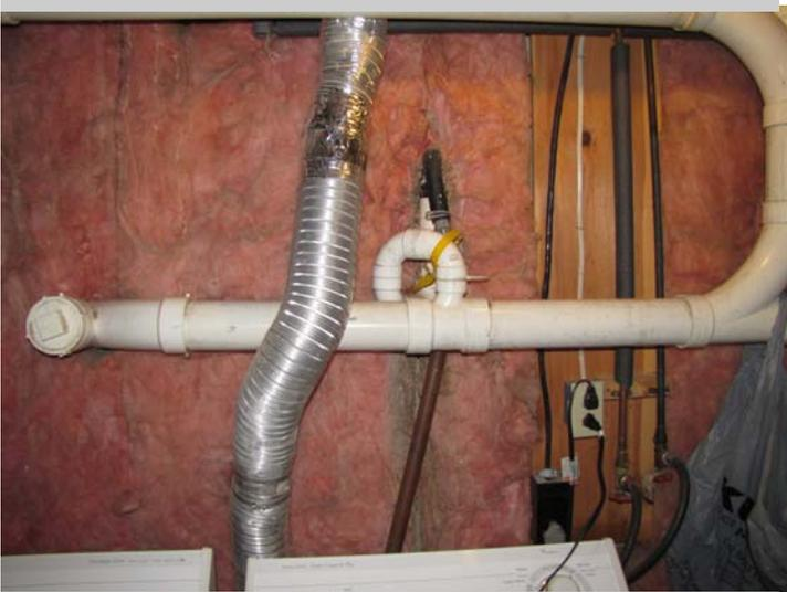
*Note the leakage behind the pipe on the insulation. This pipe is too short and will always leak.*
