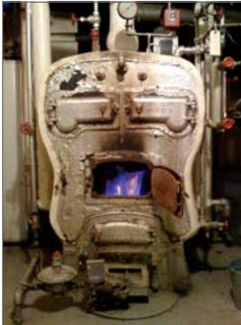
You see, trapped air is what causes short-cycling in a steam system. Most guys crank up the pressuretrol to "cure" short-cycling. That doesn't work. It just runs the fuel bill up and makes the system heat more slowly. The customer still has uneven heat, but now it costs him a lot more for the privilege. It doesn't make sense.
