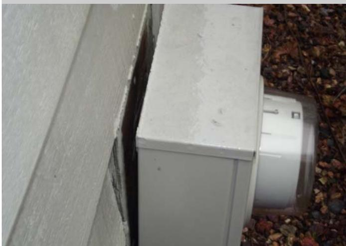
*Stress from the soil settling has pulled the meter pan away from the house, resulting in a moisture-entry point.*
