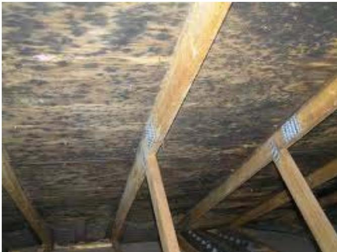
air is rising through the house, via the stack effect, that air hits a point which we refer to as the “neutral pressure plane” This is the point where the pressure in the house goes from negative (starting in the basement) to positive. Depending on how well the attic is insulated and air sealed, this will determine where that neutral pressure
